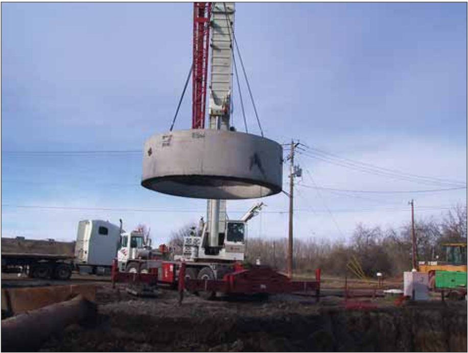
New lift station Construction crews place a huge cement pipe into the ground at the corner of 7 th Street and Nevada Avenue in Homedale last week as part of a new lift station project. City services supervisor Larry Bauer said the project is nearing completion, and he expects the station to be in operation within the next few weeks.
